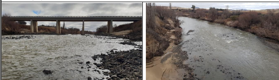
Figure 5-17: Site photographs of the Lower Caledon EWR site
